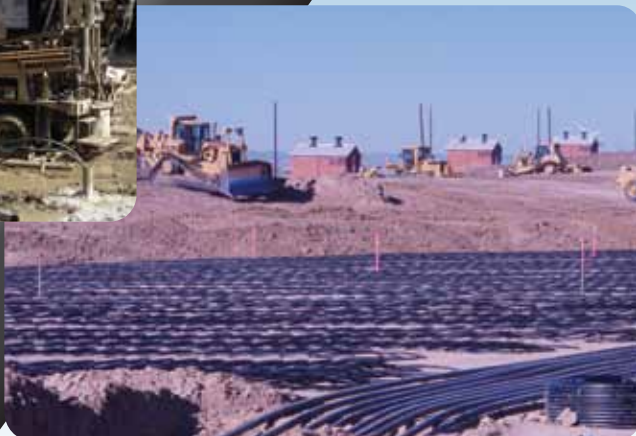
Slinky Installation
